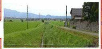
VI-2(1)西大谷川浚渫 (沖・東城寺地内)
