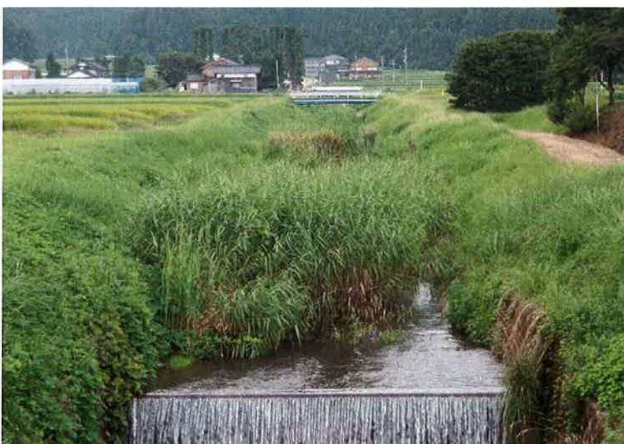
沖地内西大谷川
