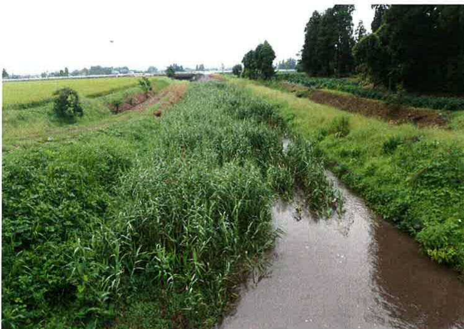
沖地内西大谷川
