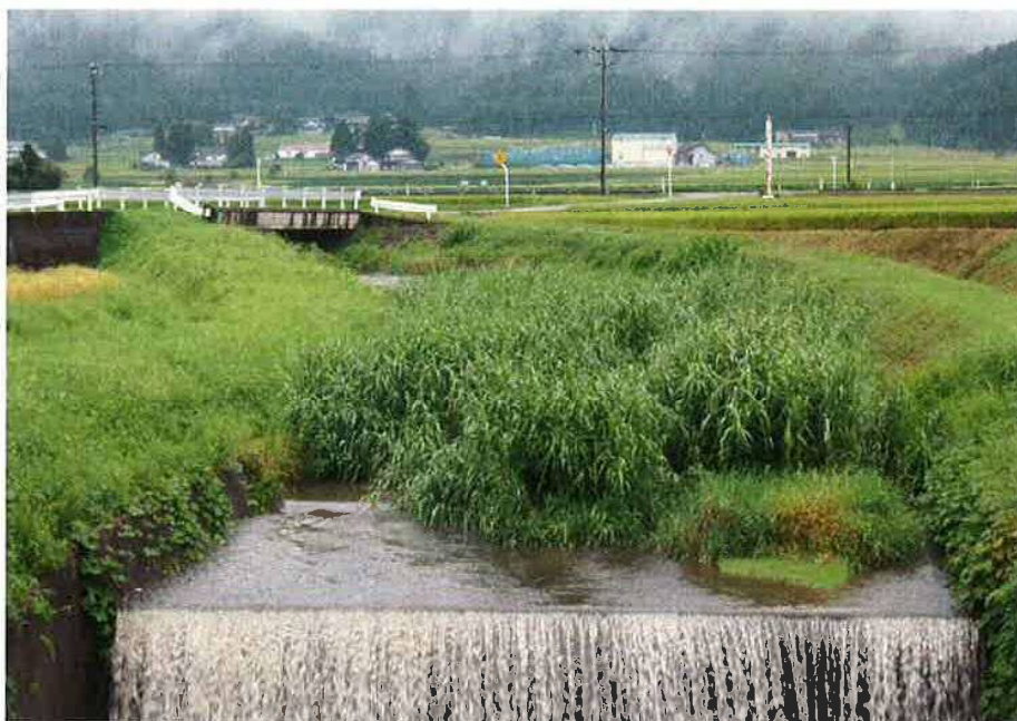
沖地内西大谷川
